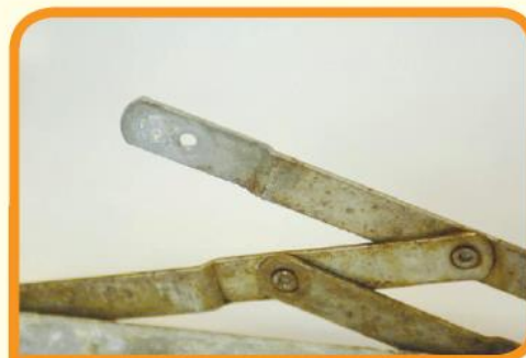
Brownish rust stain deposits on surface of the bar hinges
