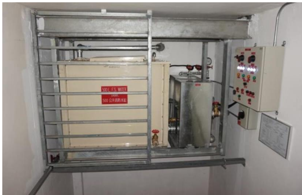
Supply Tank installed inside Roof-floor Staircase
