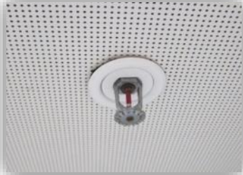
Automatic sprinkler system
