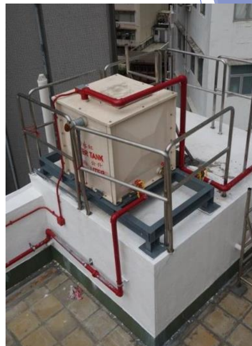
Supply Tank installed on Roof-floor
