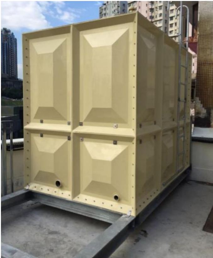
Original Supply Tank Capacity 9,000 litres
