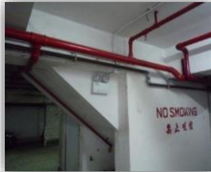
Fire hydrant and hose reel system
