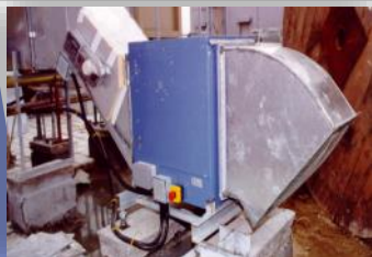
Automatic cut-off device for the mechanical ventilating system
