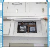
Non-emergency services (such as electric cables, meters) within staircases should be enclosed by fire barriers with adequate fire resistance rating.
